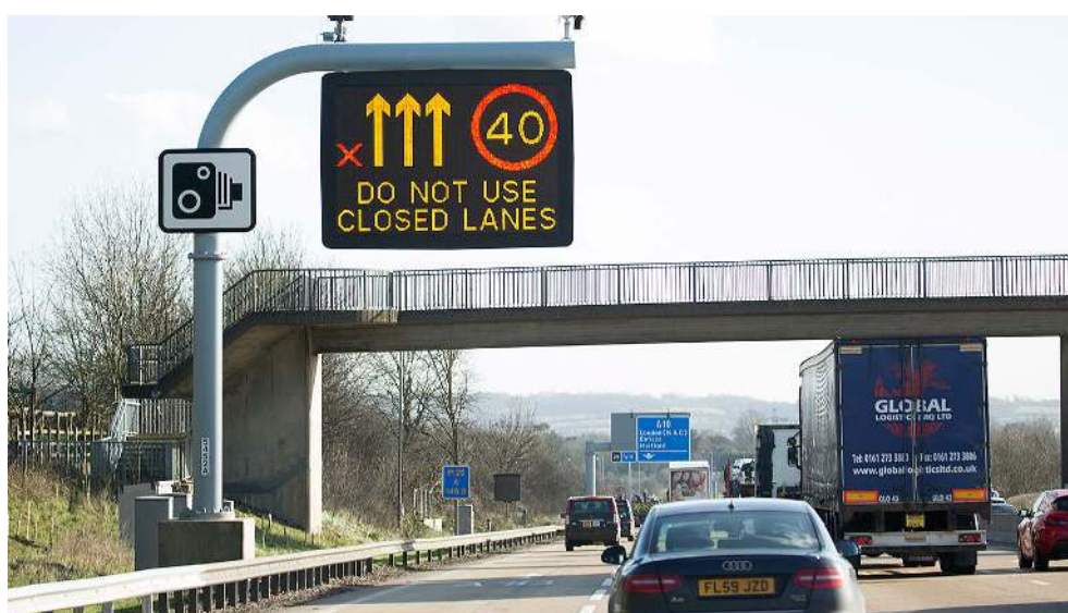
Figure 8: Smart motorway signage
